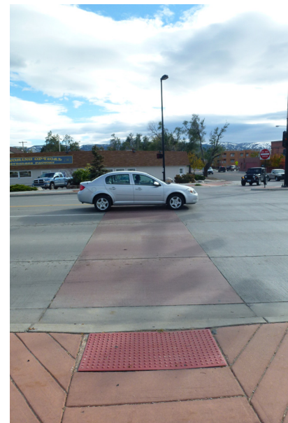
Motorists often encroach into the crosswalk area at locations where colored concrete has been used
