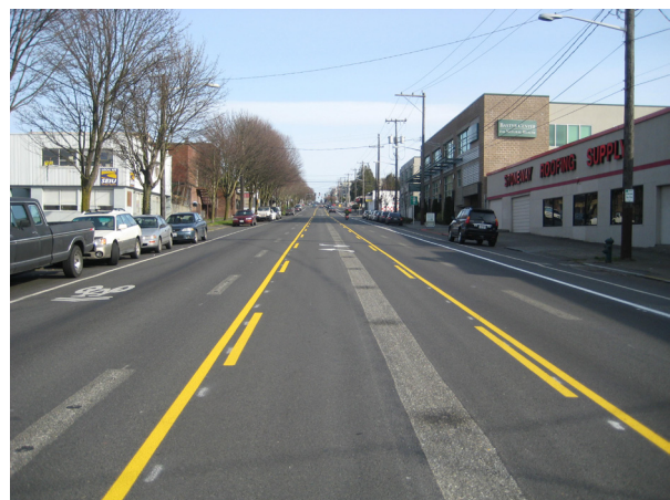
Mill markings indicate where pavement markings were removed to convert (i.e. road diet) a roadway with 4 travel lanes to 2 travel lanes with a two-way center turn lane and bike lanes.
