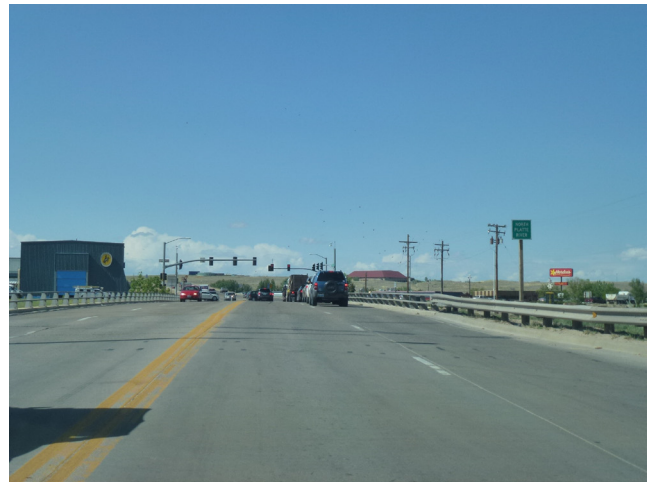
Poplar St bridges over the North Platte River and railroad are known barriers to walking and biking
