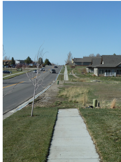
Sidewalk gaps reduce the functionality and safety of the pedestrian network
