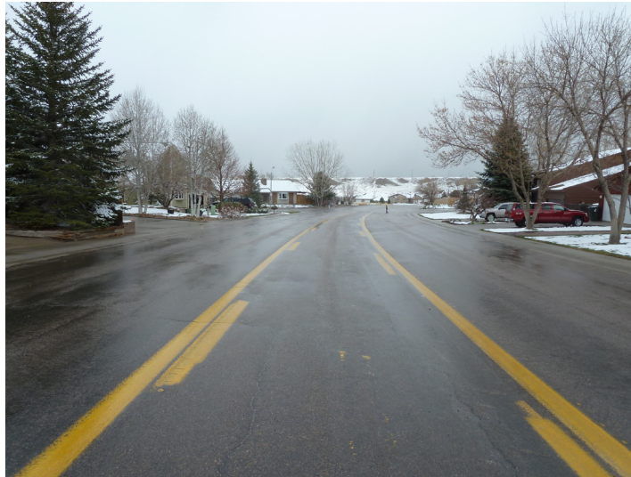
Two-way center turn lanes on streets where left-turn volumes are low provide an opportunity to reallocate roadway space and stripe bike lanes.
